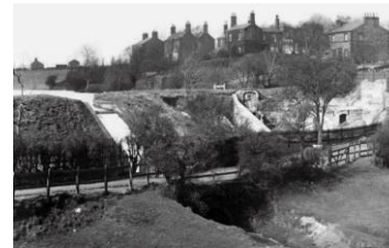
Sutton Mill Dam including the waterfall in the background. The first photograph also shows Sutton Mill in the corner. (1910)
